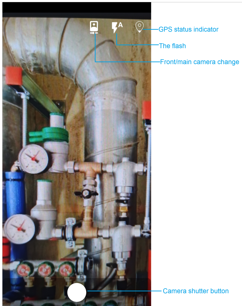
Fig. 2.25: Using the application built-in camera
